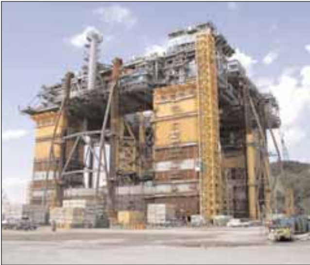
Above: Nakika platform during fit-up of the deck to the hull.
