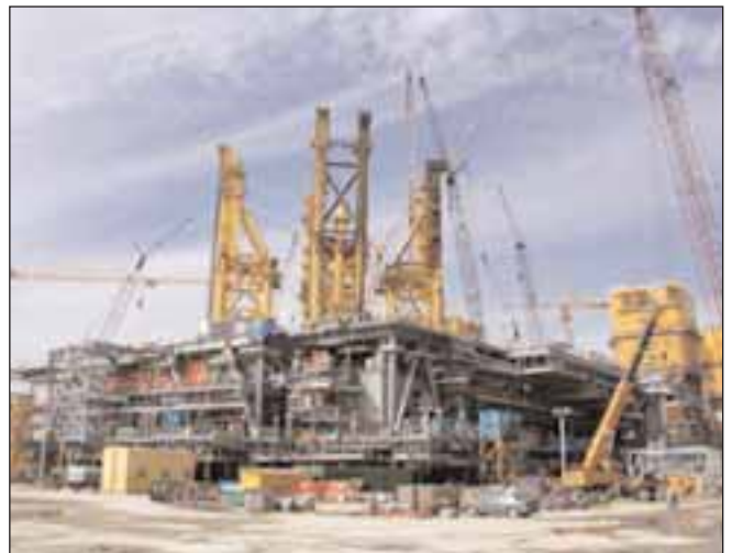
Above: The deck prior to lifting
