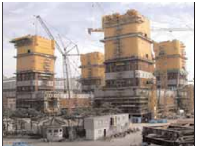
Below: The hull prior to skidding beneath the deck
