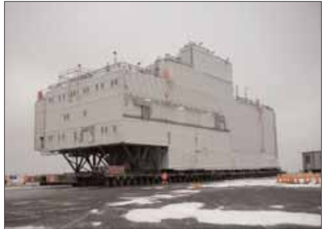
Above: Kristin L.Q. module approaching loadout quay
